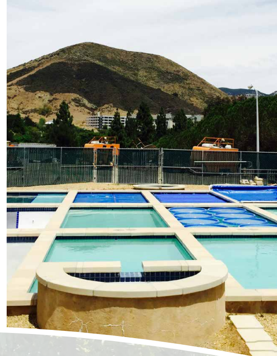
The NPC Test Pools National Pool Industry Research Center at the California Polytechnic State University - San Luis Obispo, CA
